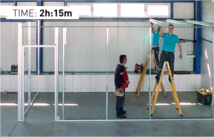
Ceiling structure assembly
