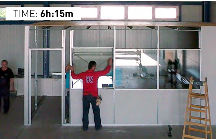
Installation of glazed panels
