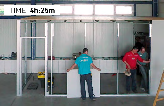
Installation of solid panels
